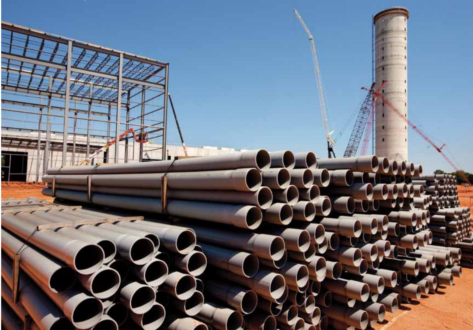
ABB: Construction of cable plant
